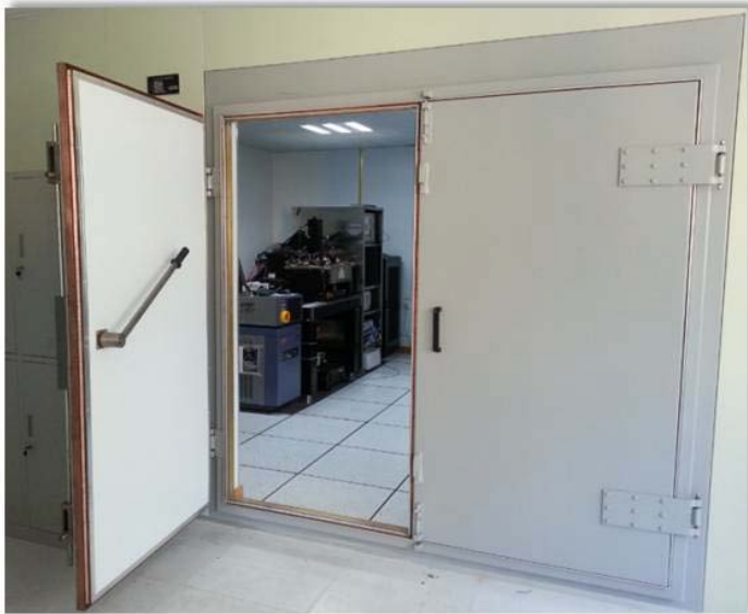
Electromagnetic shielding room
